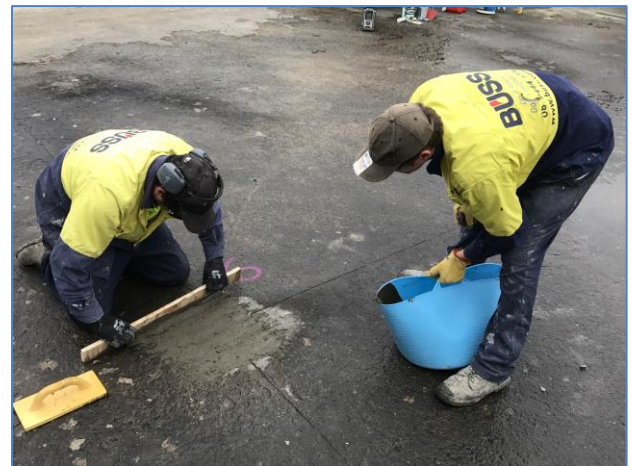
Fig.2 Repairs underway to one of multiple areas
