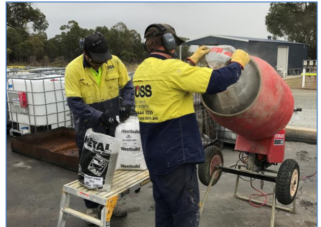
Fig.1 Preparation of bespoke heat resistant repair mortar
