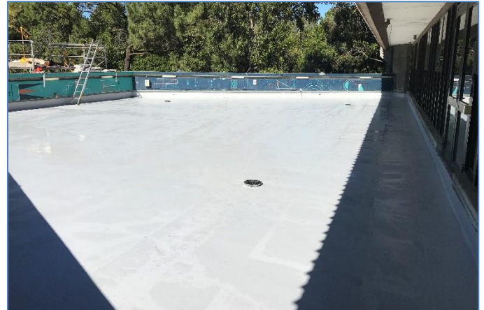
Fig.1 Completion of the five-layer waterproofing system
