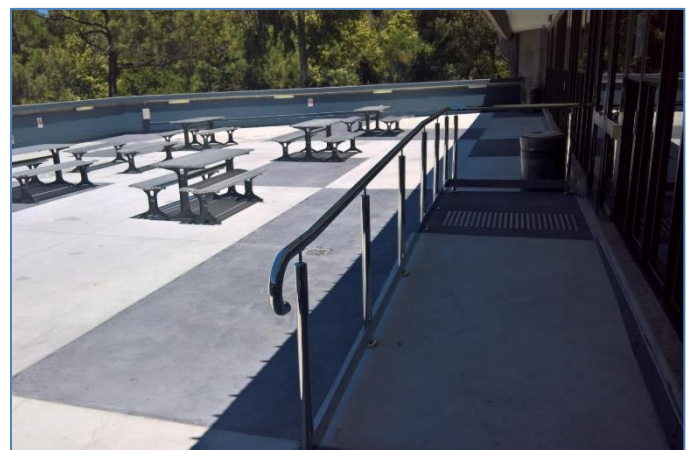
Fig.3 Newly completed deck refurbishment
