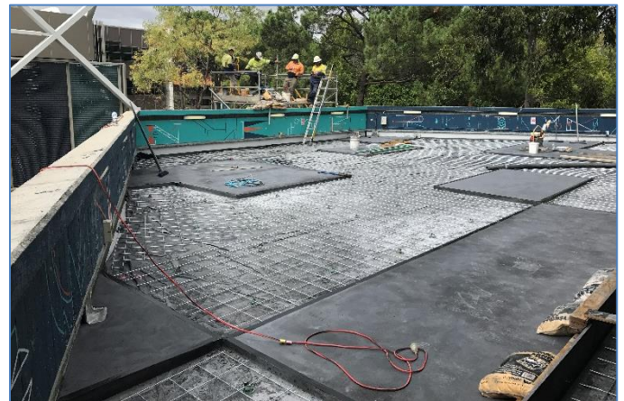
Fig.2 Concrete slabs - pour one, of two pours, completed
