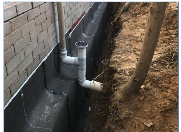
Fig.2 Waterproofing works in progress
