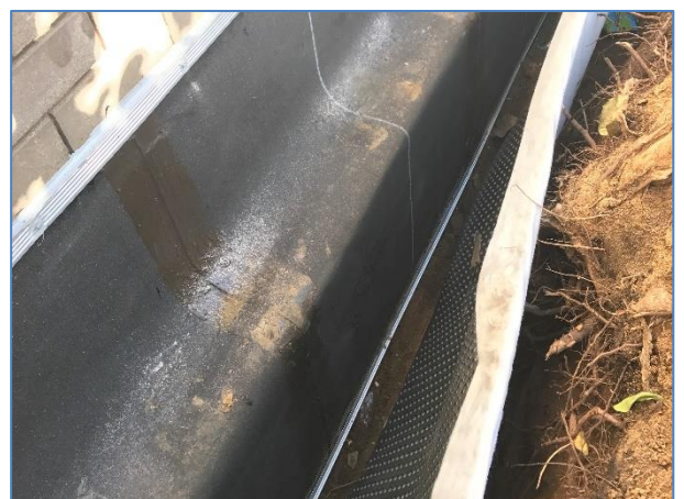
Fig.3 Two-layer waterproofing system installed
