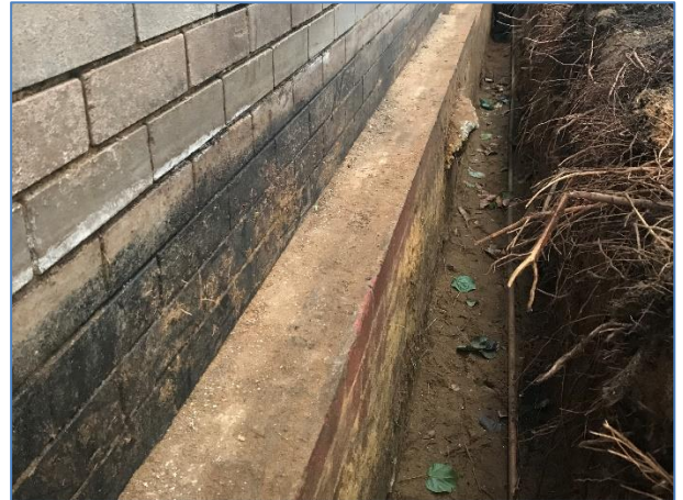
Fig.1 Excavation work underway
