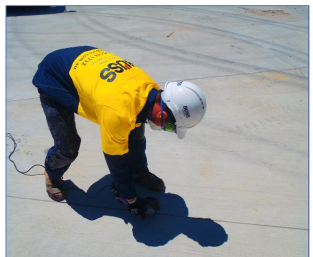
Fig.3 Concrete works commenced
