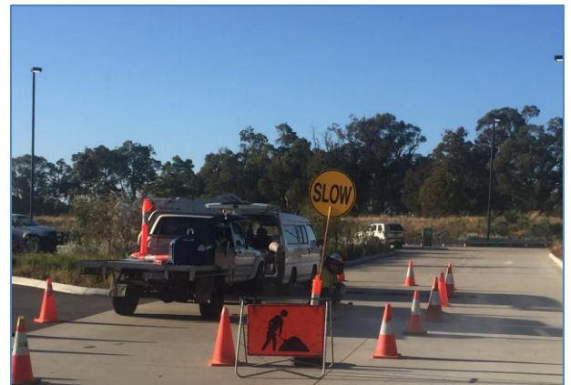
Fig.2 Traffic Management in place
