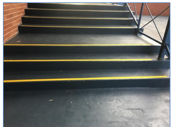
Fig.3 Hazard free stairs with uniform appearance
