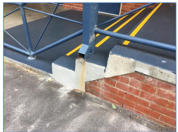
Fig.2 Repairs completed – safety hazards eliminated
