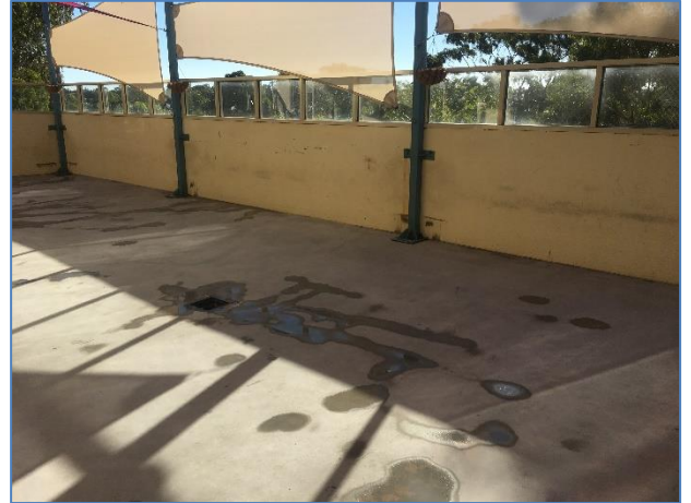
Image 1: Surface preparation in progress
