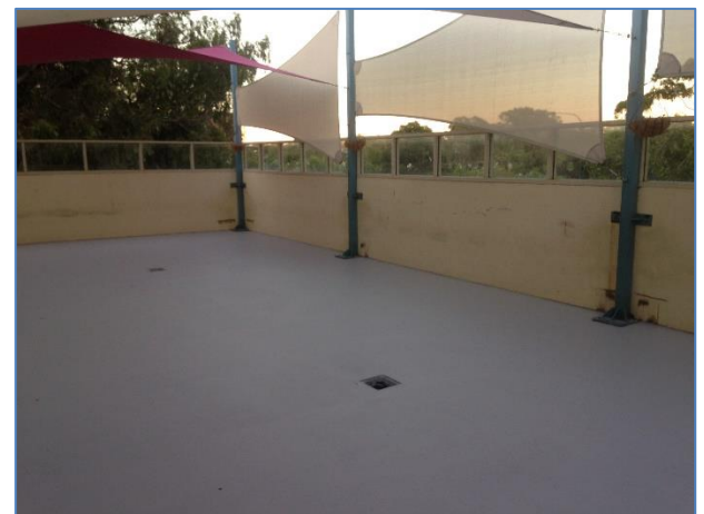
Image 3: New waterproofing membrane system
