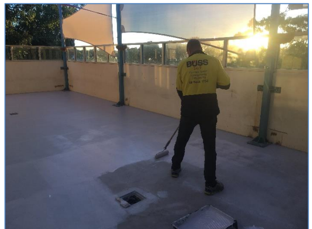
Image 2: New waterproofing membrane system being applied
