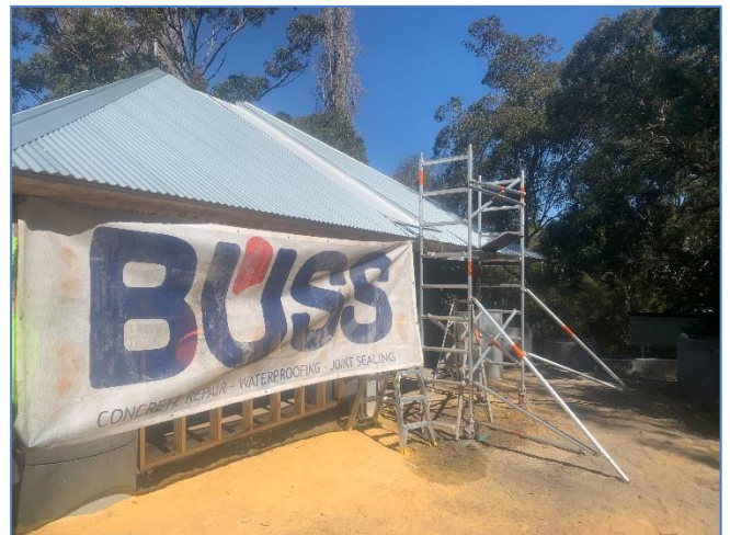
Image 2: Repairs completed – safety hazards eliminated
