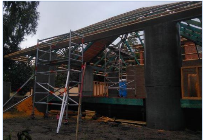
Image 1: Building under construction
