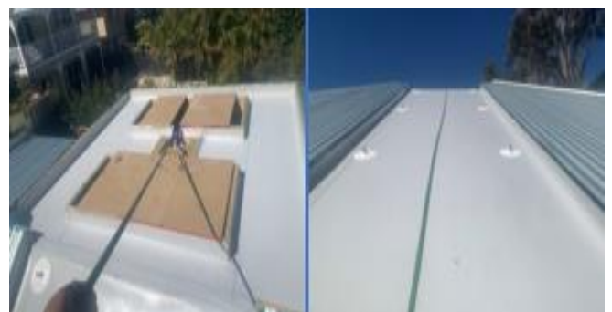
Image 3: Works completion – seamless finish to rooftop and roof pitch
