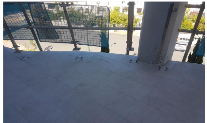
Fig.3 Completion of tiling and welding of balustrade bolts
