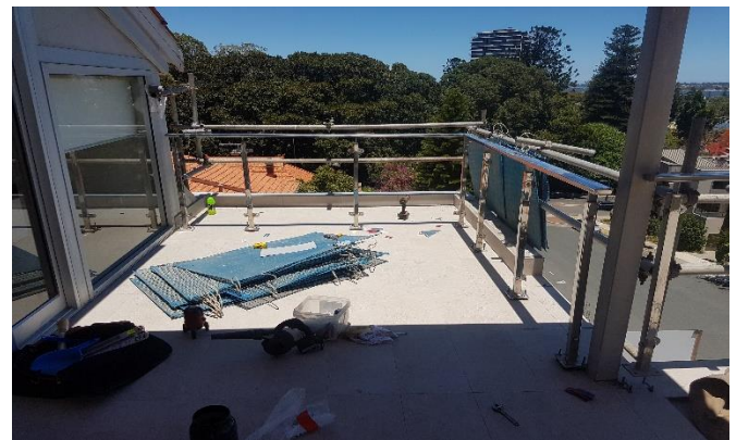
Fig.2 Tiling and balustrade installation in progress
