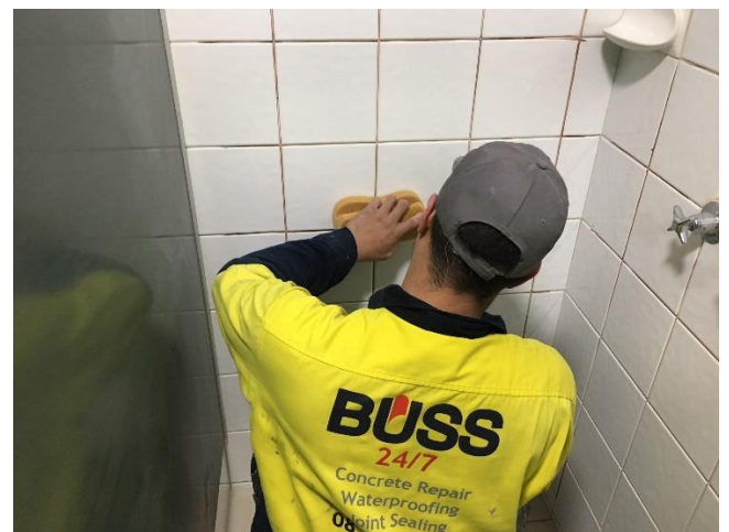
Fig.3 Grouting works in progress
