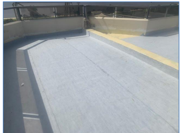
Image 2: Works nearing completion
