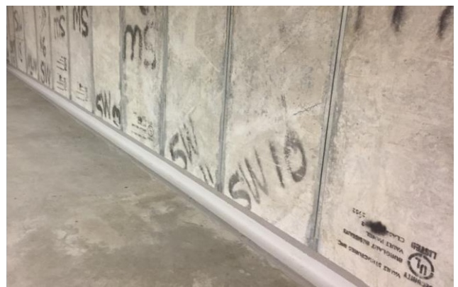
Image 3: Vault area upon works completion
