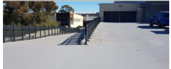
Image 2: Door 1 entrance – before and after
