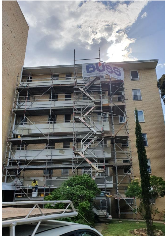
Image 1: Remedial works to the balcony upstands in progress
