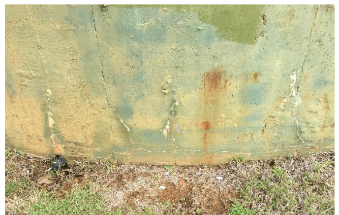
Image 3: Defective concrete
