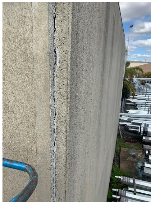
Image 2: Before joint sealant
