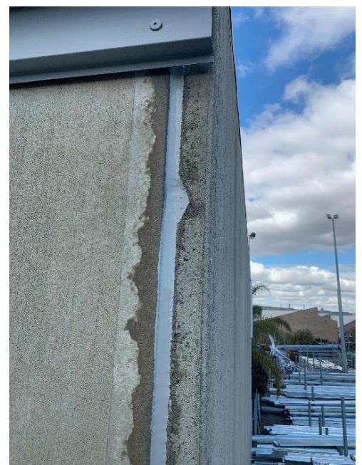
Image 3: After joint sealant
