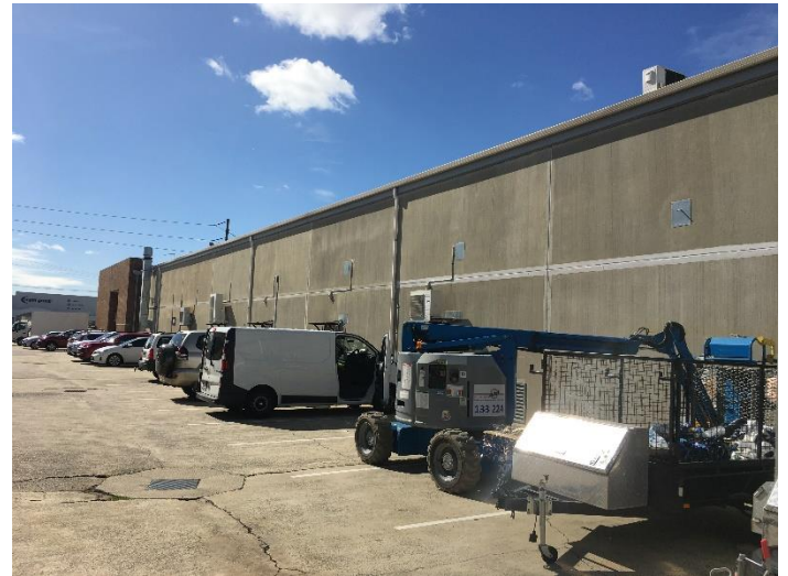
Image 1: Concrete panels to rear of the building
