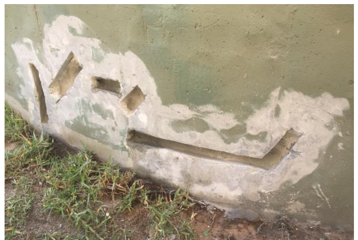
Image 3: Preparation works for a repair area
