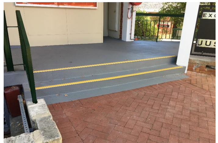
Image 3: Repairs & coatings works at completion
