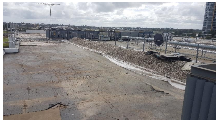
Image 2: Surface preparation works underway
