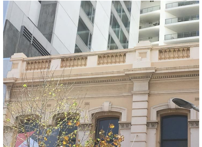
Image 1: 92 Barrack Street upper floor balustrade
