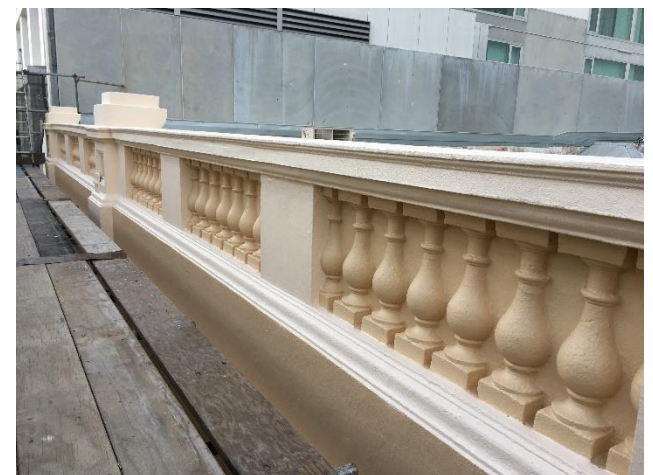
Image 3: Repairs completed; balustrade
