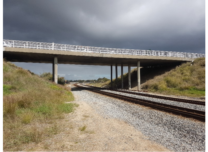
Image 1: Bridge 1137 over S.G. Railway
