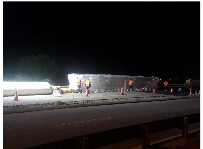
Image 2: Establishment of work site
