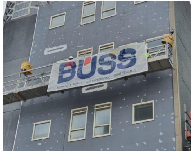
Image 2: Access system installed & structural assessment undertaken
