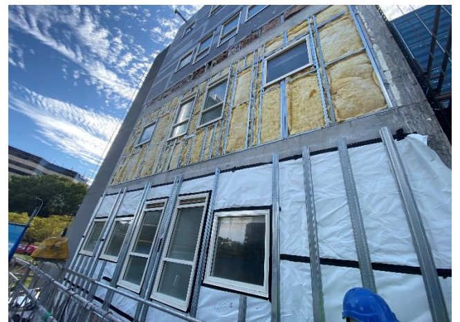
Image 3: Installation of new insulation & sarking
