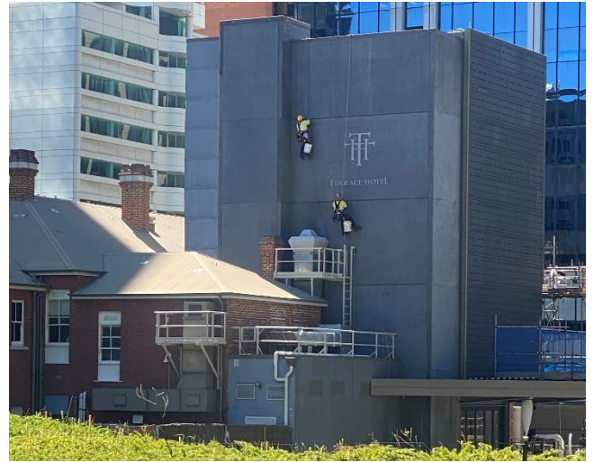
Image 1: Panel joint replacement in progress
