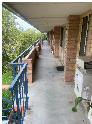
Image 4: Before walkway coating
