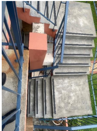
Image 2: Before – stairwell coating
