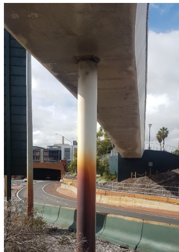
Image 3: Prior to works
