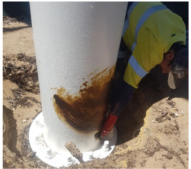
Image 2: Bridge pier Denso wrapping in progress
