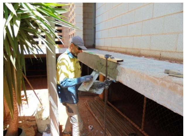
Image 4: Concrete repairs ongoing to external soffit area
