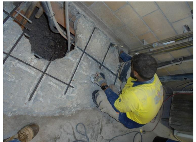
Image 3: Repairs to plantroom floor in progress
