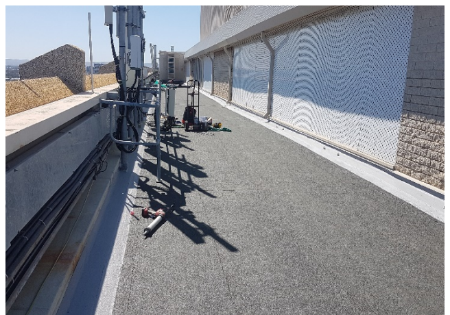
Image 3: Waterproofing works in progress
