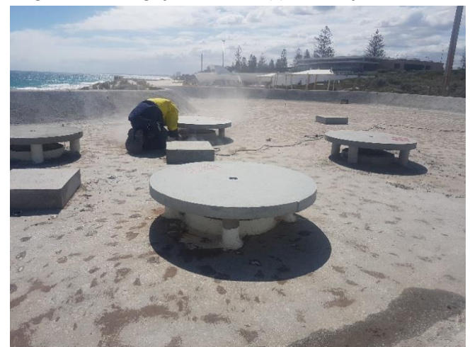
Image 3: Replacement of concrete discs over roof breathing vents
