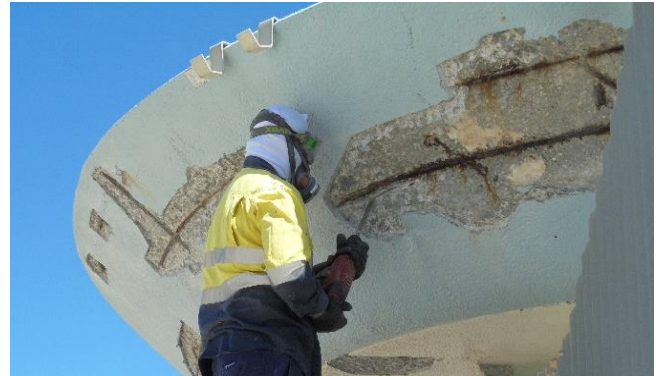
Image 1: Concrete breakout works to soffit
