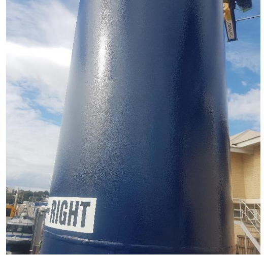
Image 1: Jetty crane to be blasted & painted
