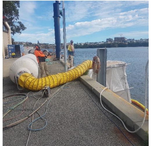
Image 2: Dust extraction & filter system for blasting & painting
