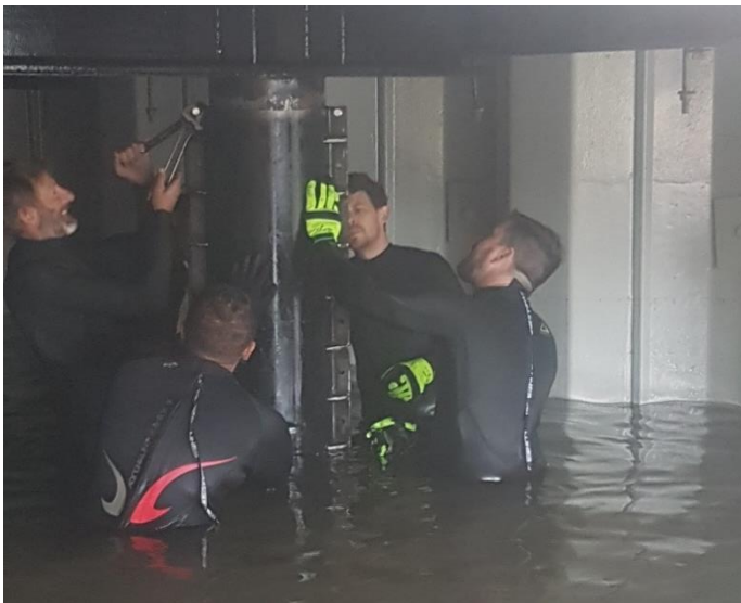
Image 7: Pile sleeve installation in progress
