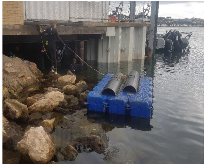
Image 6: A pontoon was used to float the pile sleeves under wharf
