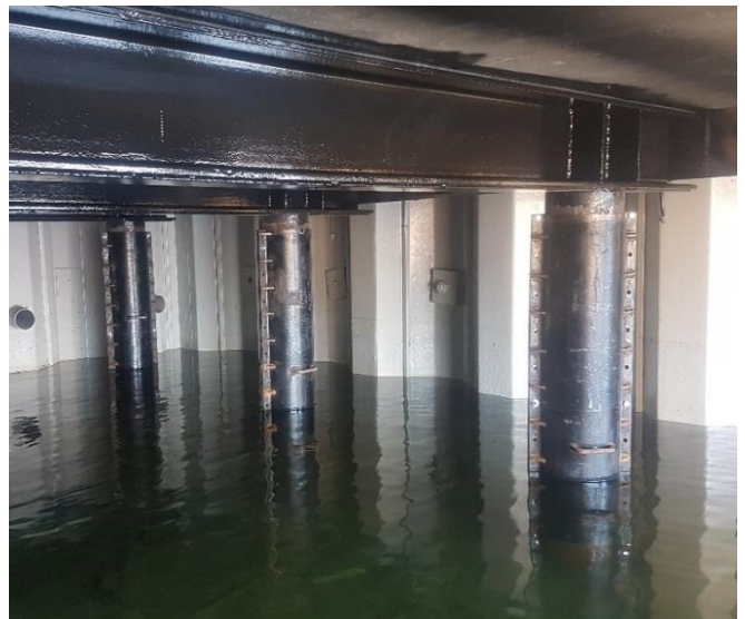
Image 8: Pile sleeve installation complete
