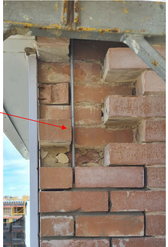
Image 4: Reconstruction of wall nib bricks around new roof tie-down
