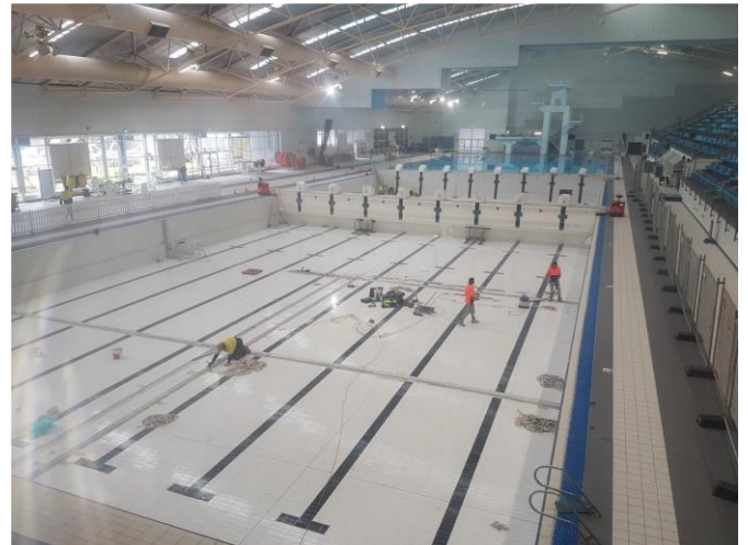
Image 2: Removal of joint material
