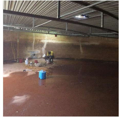
Image 1: Works to internal of tank in progress
