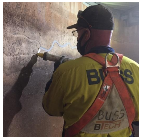
Image 3: Joint sealing works in progress
