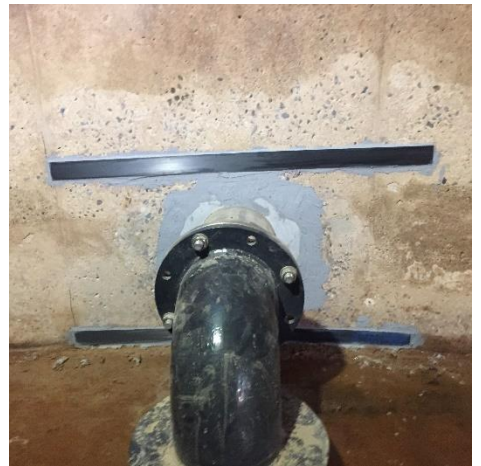
Image 2: Installation of new outlet/inlet complete
