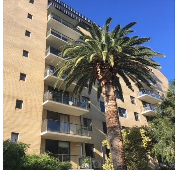
Image 1: Western façade of Riverview Apartments
