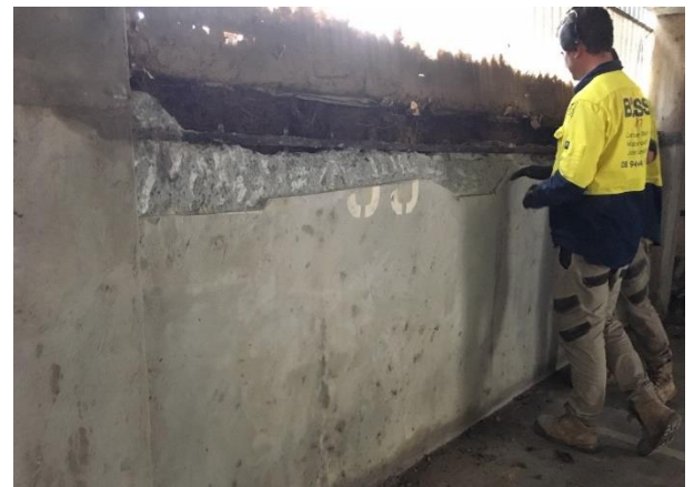
Image 3: Concrete repairs to undercover carpark
