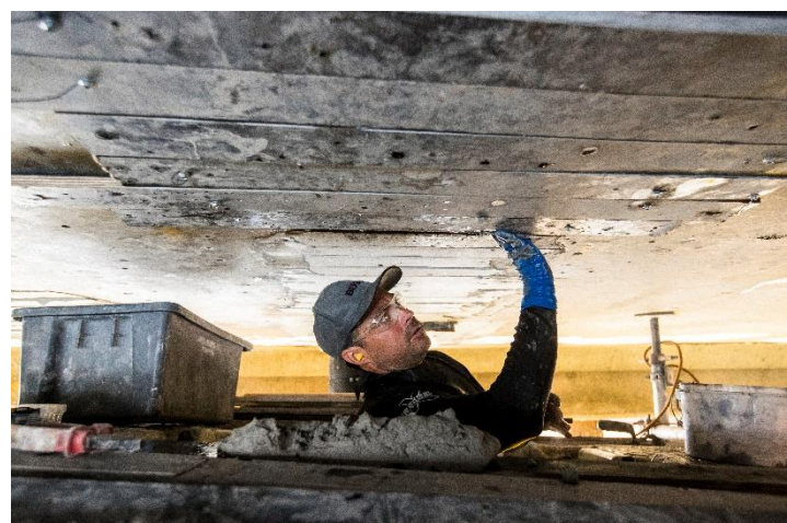
Image 3: Concrete repairs in progress
