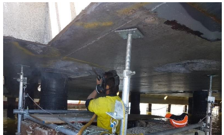
Image 2: Concrete breakout works in progress via specialised access system
