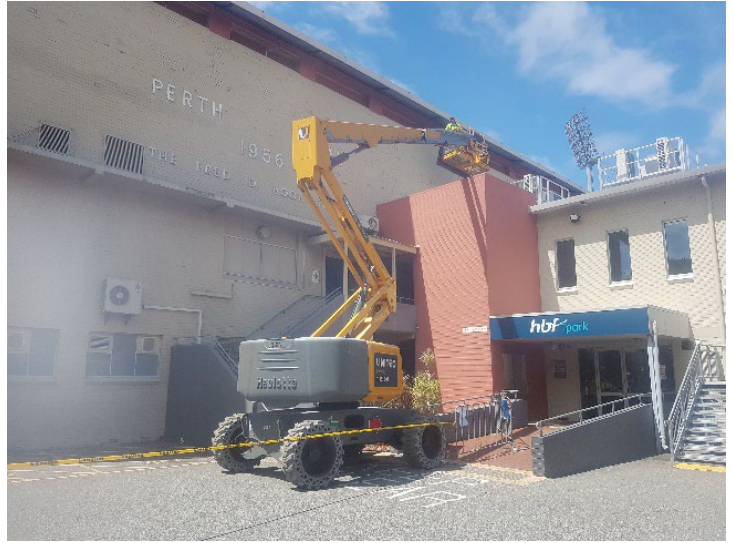
Image 1: Repairs to external brickwork in progress
