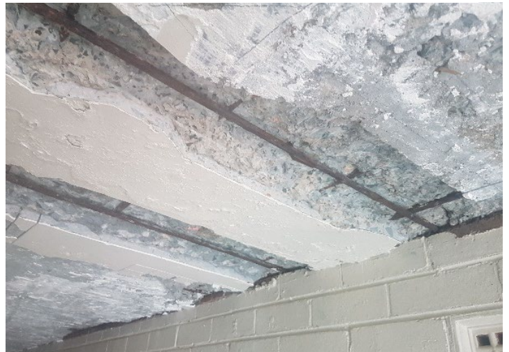
Image 2: Concrete breakout to tunnel ceiling
